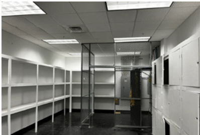
Storage, Electric & Data Room
